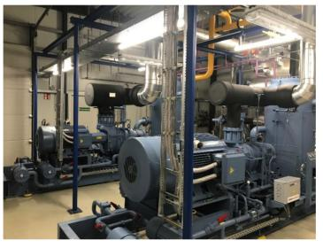
The SRMTec combination of 1 x SRM26M and 1 x SRM20M compressor-pack as booster system assures a maximum of flexibility with several side loads and is ready for future extensions.
