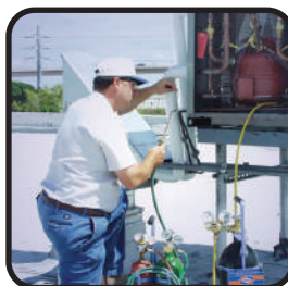
Purge and pressure test an A/C&R system
