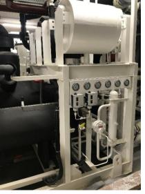
Dry-Coolers and high efficient Plate in Shell Condensers and Evaporators with integrated phase-separation domes were used to reduce the refrigerant to a bare minimum of xxx kg.
