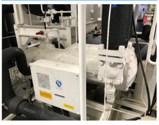
The system is operating in summer mode for cooling and can be switched over easily to wintre mode for heating In winter operation the Ammonia receiver is acting as an economizer to
