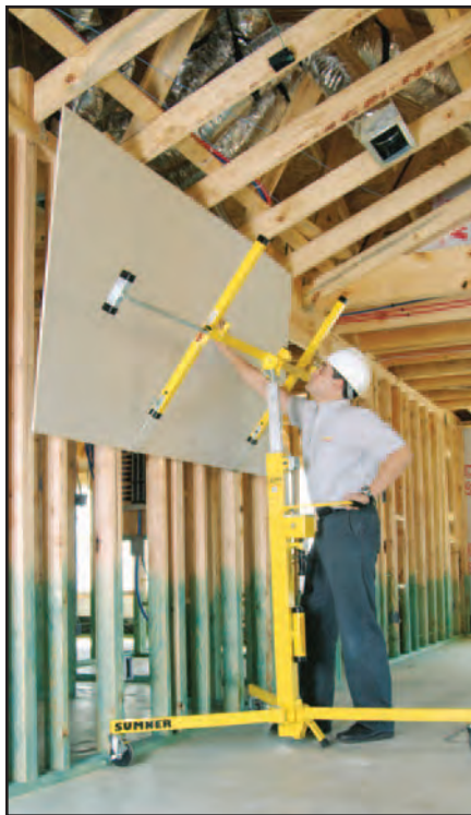
Steering leveler provides optimum positioning.
